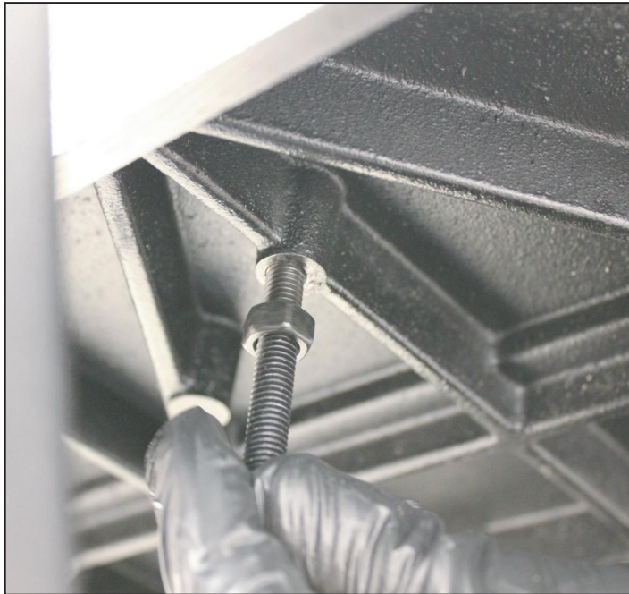
Figure 9: Installing the 90-degree table stop.
